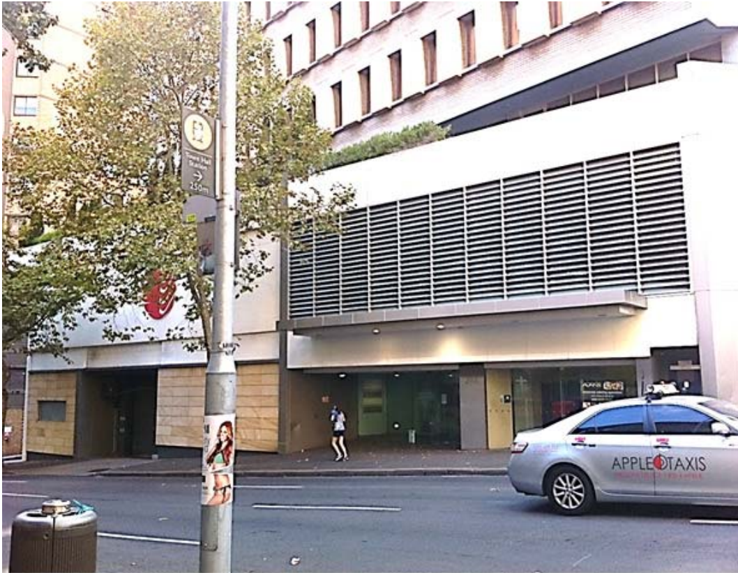
Figure 5: The existing ground floor retail and vehicular access to the site on its Sussex Street frontage.
