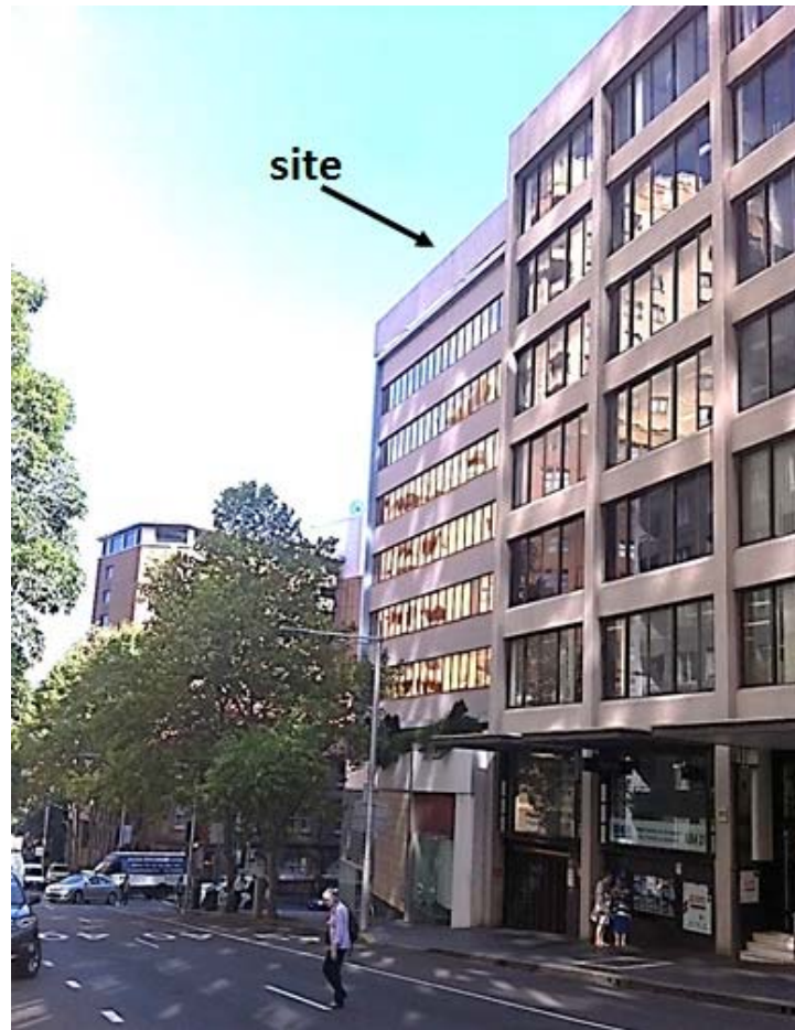
Figure 3: The site as viewed from Bathurst Street looking west.
